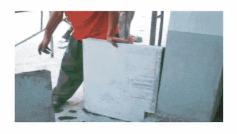
4. Installation: Carrying the board prepared to be installed to the installation place, correcting the wall board by gavelock and making it close tightly, and let the polymer mortar squeeze out into full and fixing it with a chock temporarily.
