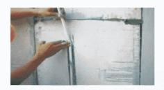
8. Installing electrical wires and switches: Setting lines on the places needing to be set with concealed wire and switch box, then cut a groove by handhold electric saw, filling with polymer mortar after installation.
