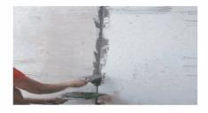
6. Grouting and filling starch: Filling and strickling the corrected wall board with polymer mortar, filling the big gap with pea gravel concrete.
