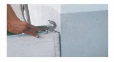
5. Correcting, fixing: Using a guiding rule of two meters or longer to check verticality and leveling correction, then using  $\Phi$  6mm or  $\Phi$  8mm reinforcing steel bar with ribs adding with construction sealant to fix.
